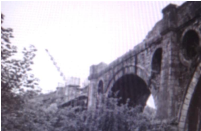
Rebuilding work in progress during 1962
